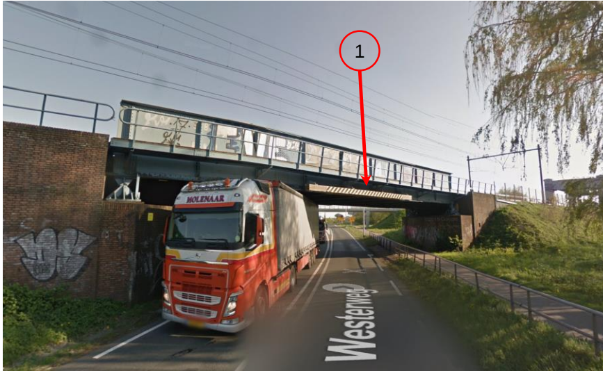
Steel bridge over the N242 near Heerhugowaard
